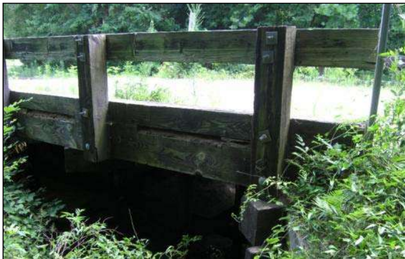
Photo 5-23. Hill Road over Little Mills Creek, Nassau County (No. 744006)
