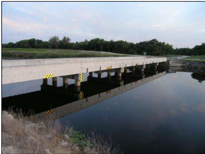
Photo 5-22. CR-721A over Harney Pond Canal, Glades County (No. 054015)
