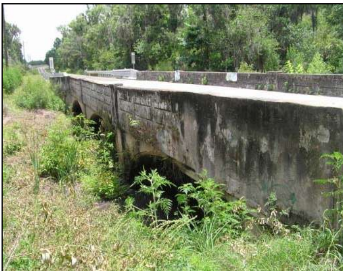
Photo 5-7. Little Payne Creek Bridge, Hardee County (No. 060034)
