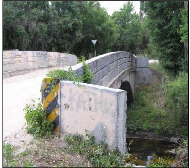
Photo 5-8. Payne Creek Bridge, Hardee County (No. 064069)
