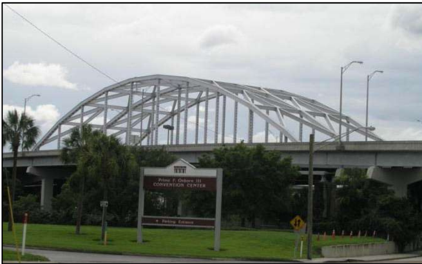
Photo 5-9. Myrtle Avenue Overpass, Duval County (No. 720163)
