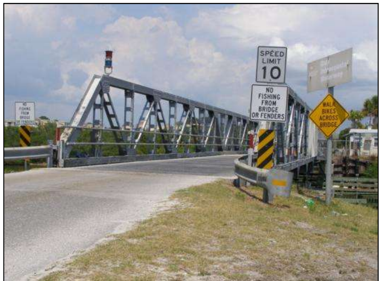
Photo 5-56. Blackburn Point Swing Bridge, Sarasota County (No. 170064)
