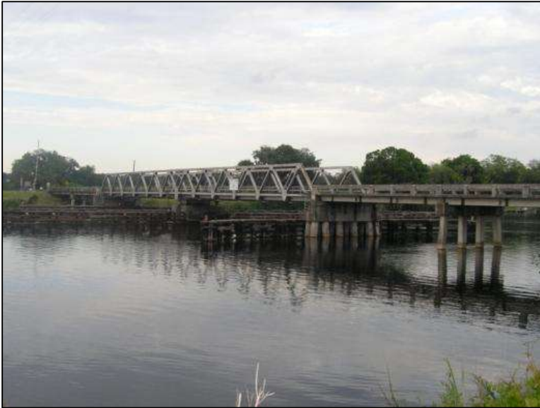
Photo 5-55. Ft. Denaud Swing Bridge, Hendry County (No. 070013)
