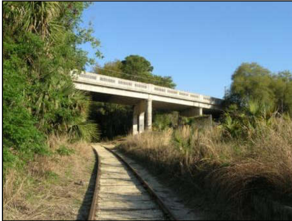
Photo 6-23. Mt. Dora Overpass/Highland Street Bridge, Lake County (No. 114089)
