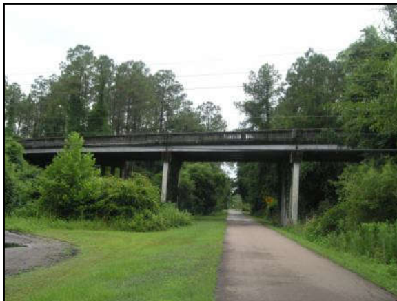
Photo 6-25. 1940 Baldwin Overpass, Duval County (No. 720026)
