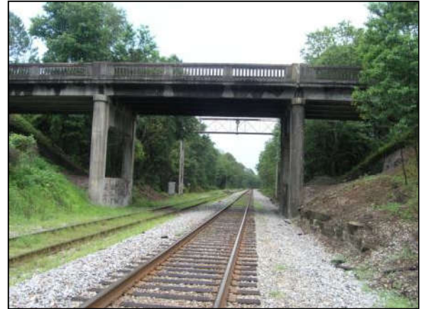
Photo 6-24. US-301/SR-200 over SCL RR, Nassau County (No. 740022)
