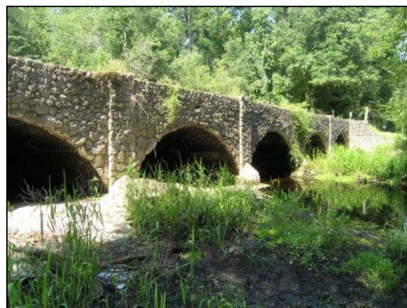
Photo 6-22. 164 th Street / Little Creek Culvert, Suwannee County (No. 370004)
