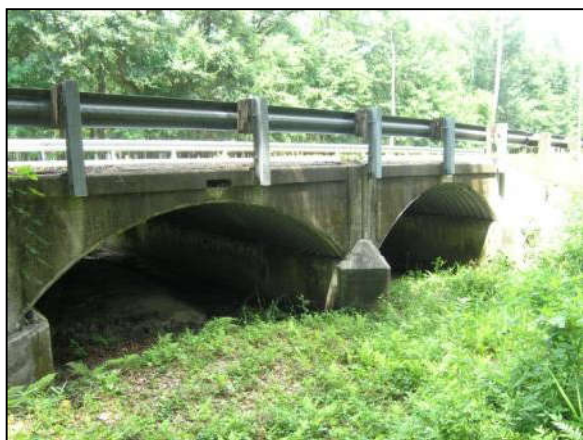
Photo 6-21. CR-18/Sampson River Branch Culvert, Bradford County (No. 280038)
