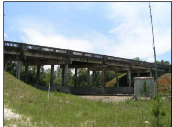
Photo 6-26. 1936 Sanderson Overpass, Baker County (No. 270001)
