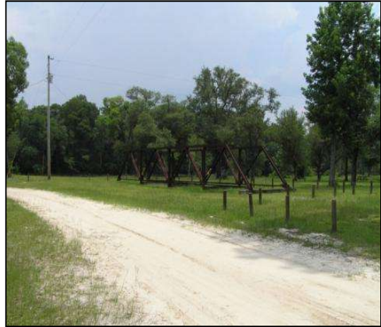
Photo 7-10. Current Location of Log Lake Bridge Remains (June 2010).
