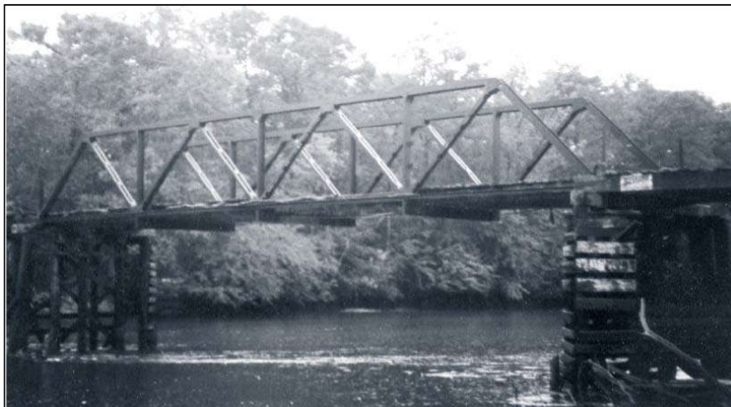
Photo 7-8. Historic View of the Log Lake Truss Bridge.
