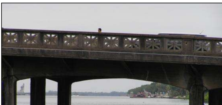
Photo 5-79. Detail of Eight-Point Star Railing Decoration.
