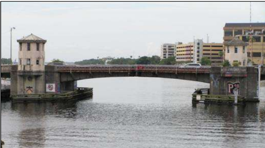
Photo 5-78. Platt Street Bridge, Hillsborough County (No. 105500)
