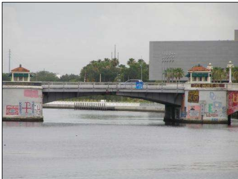
Photo 5-77. Kennedy Boulevard Bridge, Hillsborough County (No. 100100)
