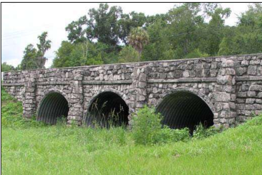
Photo 5-50. Blackwater Creek Relief Structure, Hillsborough County (No. 100647)
