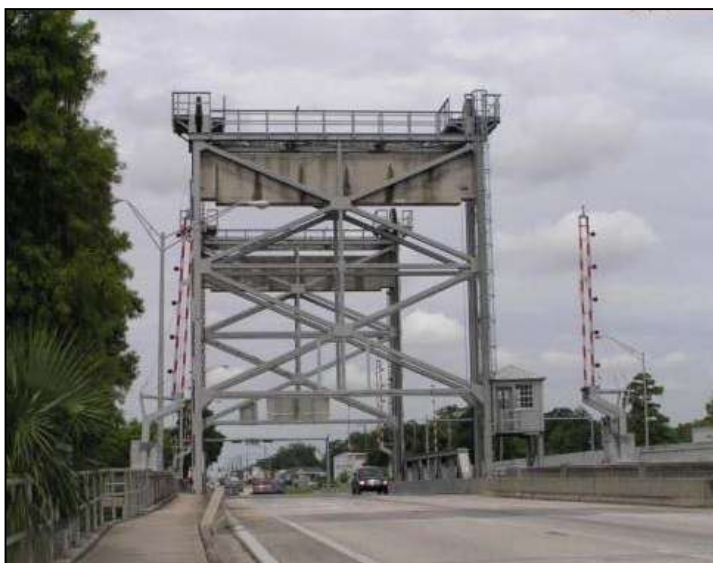
Photo 5-54. Hillsborough River Lift Bridge, Hillsborough County (No. 100920)
