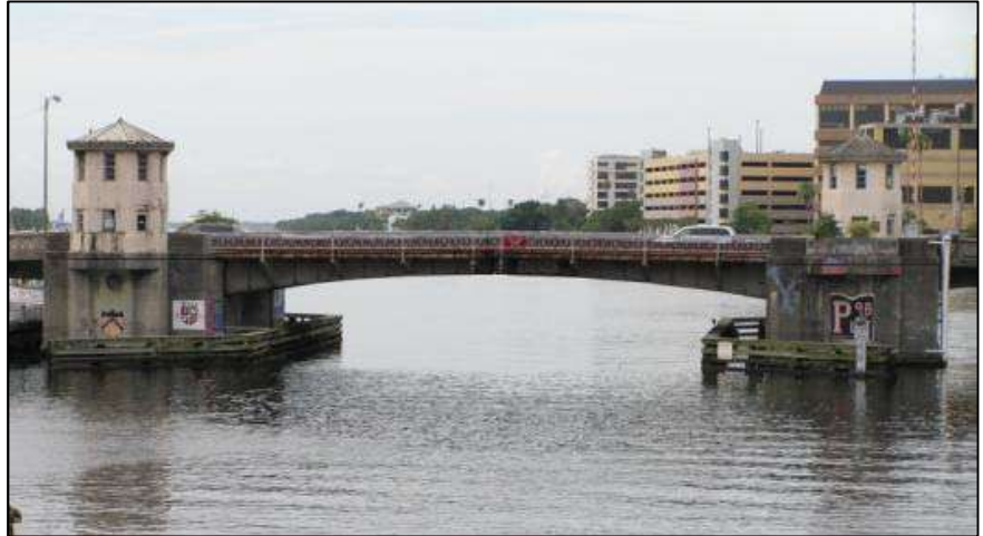
Photo 5-78. Platt Street Bridge, Hillsborough County (No. 105500)
