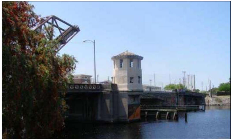
Photo 5-80. Cass Street Bridge, Hillsborough County (No. 105502)
