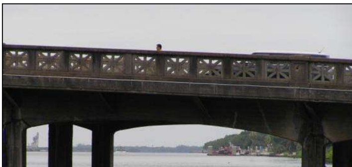
Photo 5-79. Detail of Eight-Point Star Railing Decoration.
