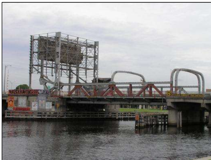
Photo 5-81. Laurel Street Bridge, Hillsborough County (No. 105503)
