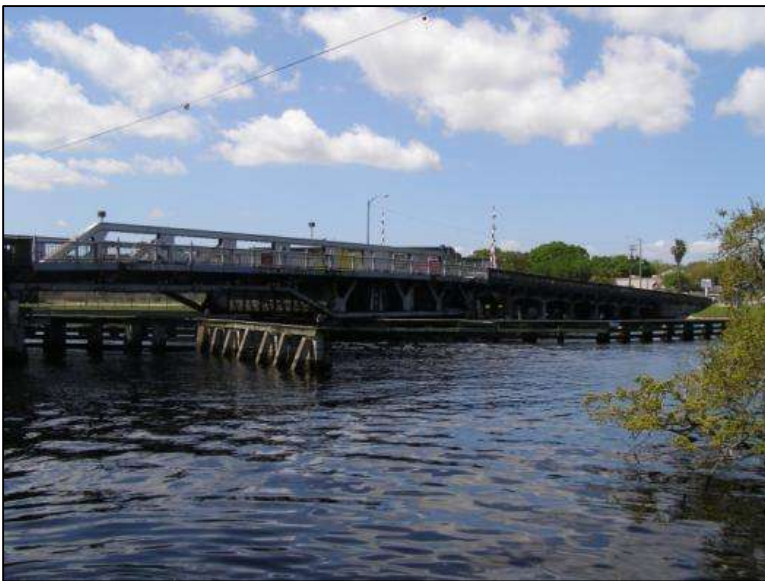
Photo 5-64. Columbus Drive Swing Bridge, Hillsborough County (No. 105504)
