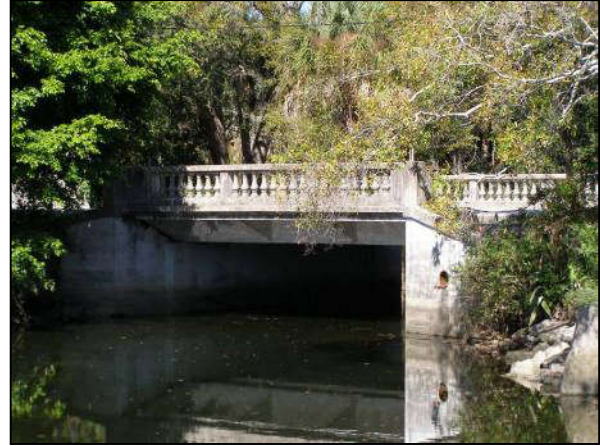
Photo 6-16. South elevation of the Twelfth Avenue Bridge, Looking Northwest.
