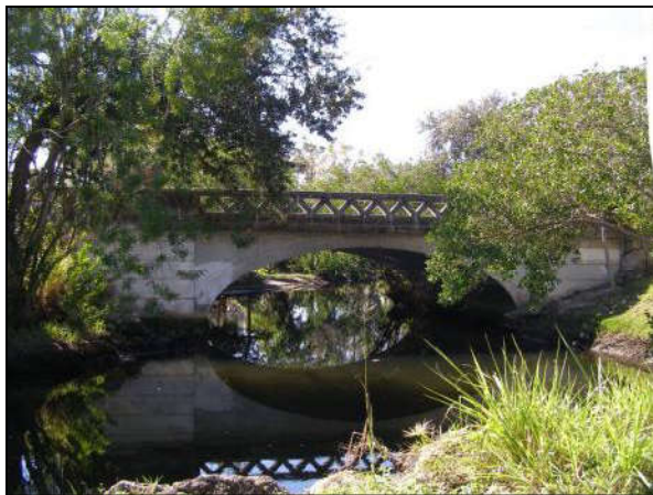
Photo 6-17. The Ninth Avenue Bridge (No. 135251), Looking Southwest.
