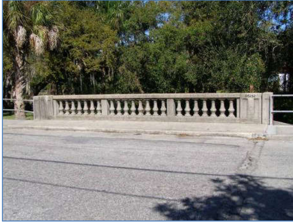
Photo 6-15. North Guardrail and Deck of the Twelfth Avenue Bridge (No. 135252)
