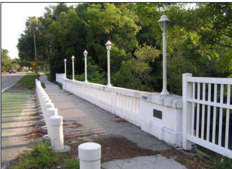
Photo 5-18. Philippe Parkway Bridge, Pinellas County (No. 150009)
