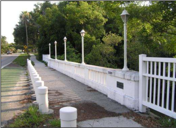
Photo 5-18. Philippe Parkway Bridge, Pinellas County (No. 150009)
