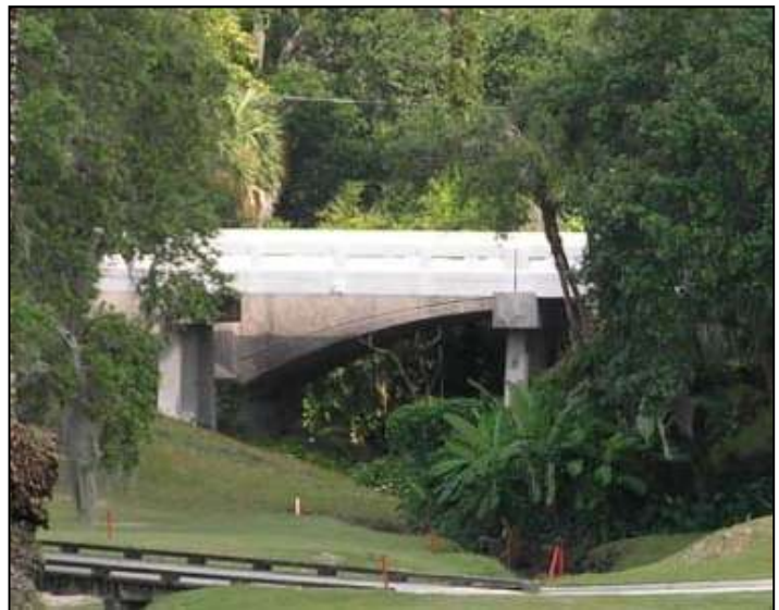
Photo 5-20. Luten “Half-Arch” Bridge, Pinellas County (No. 159901)
