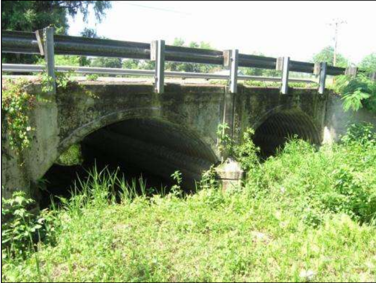
Photo 5-48. CR-18 over Braggs Branch, Bradford County (No. 280036)
