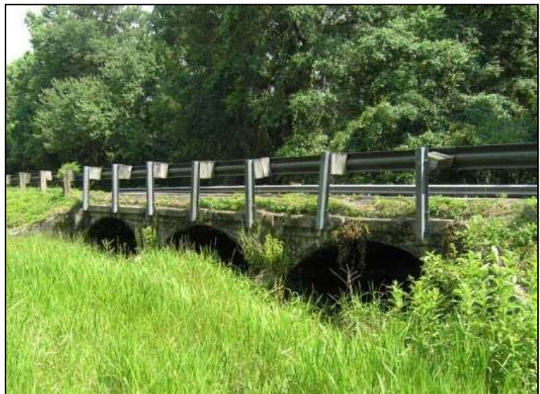
Photo 5-49. CR-18 over Gum Creek, Bradford County (No. 280037)
