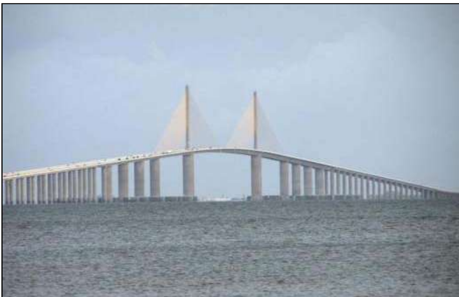
Photo 5-47. Bob Graham Sunshine Skyway Bridge (No. 150189)
