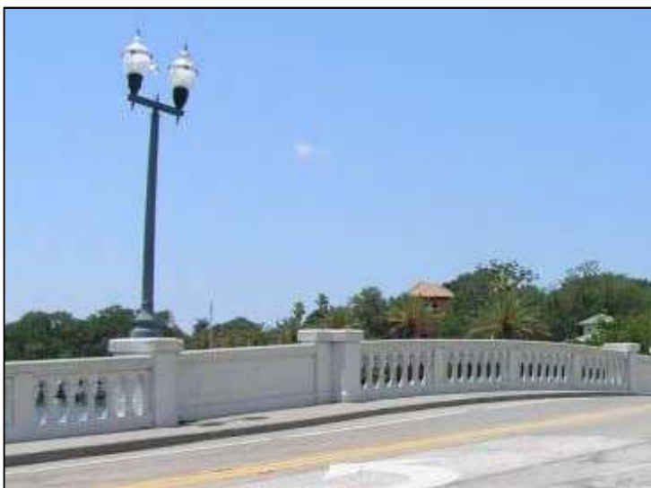
Photo 5-34. Snell Isle Bridge, Pinellas County (No. 157191)
