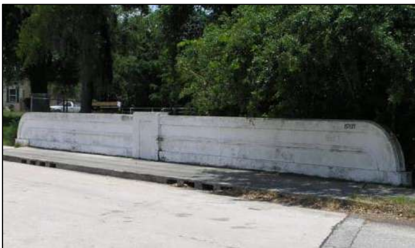
Photo 5-35. Burlington Avenue Bridge, Pinellas County (No. 157127)
