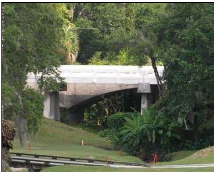
Photo 5-20. Luten “Half-Arch” Bridge, Pinellas County (No. 159901)
