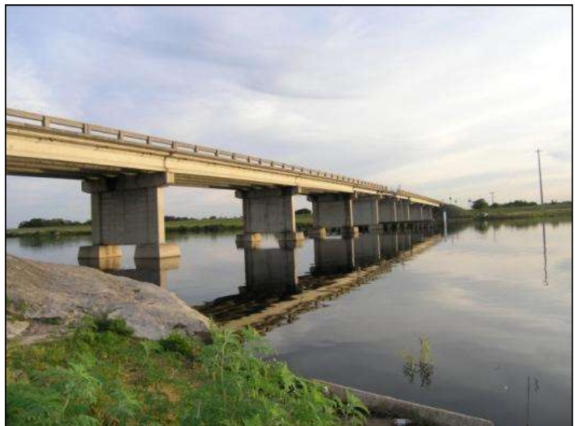
Photo 5-38. SR-78 Bridge, Okeechobee County (No. 910009)
