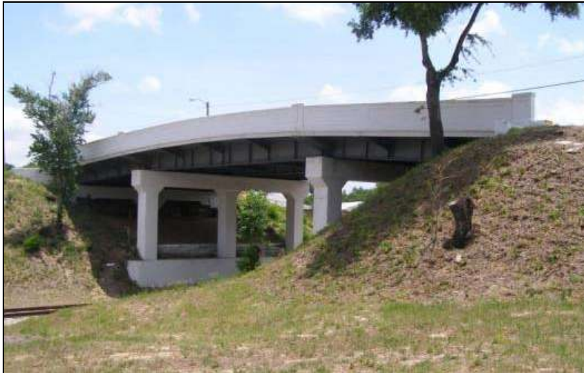
Photo 5-37. Haines City Overpass, Polk County (No. 165700)
