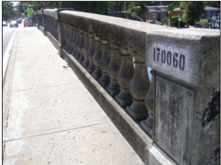
Photo 5-26. Hanson Bayou Bridge, Sarasota County (No. 170060)
