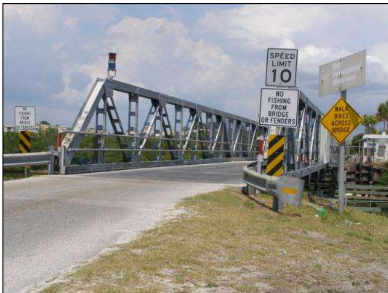
Photo 5-56. Blackburn Point Swing Bridge, Sarasota County (No. 170064)
