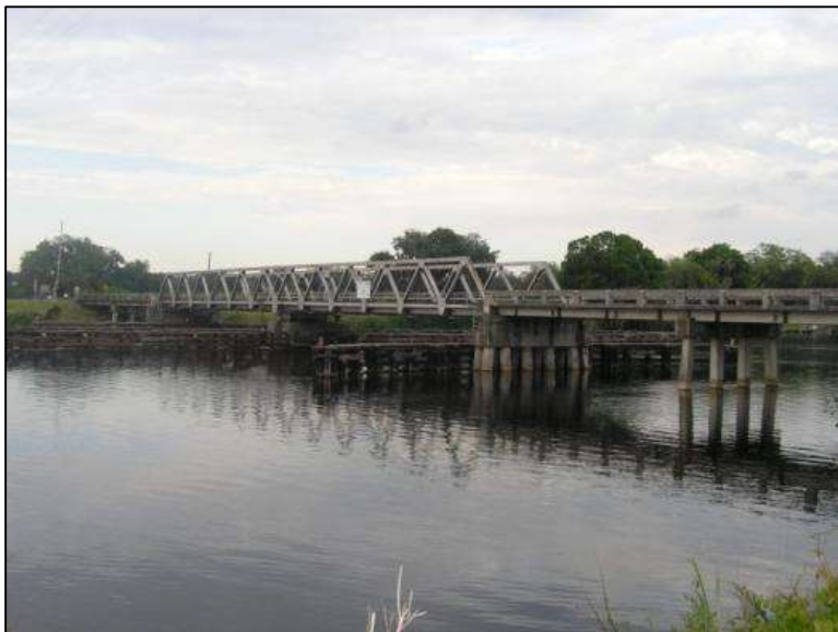
Photo 5-55. Ft. Denaud Swing Bridge, Hendry County (No. 070013)
