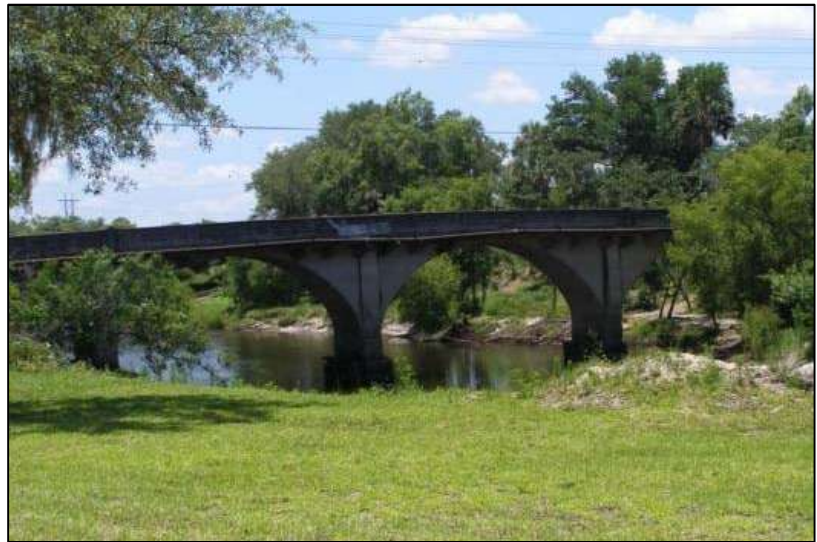
Photo 5-5. Peace River Bridge at Arcadia, DeSoto County (No. 450001)
