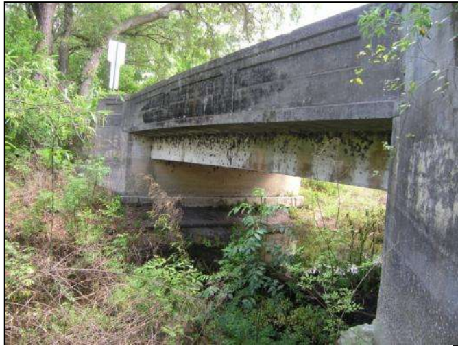
Photo 7-5. Big Prairie Canal Bridge, Sumter County (No. 184000).
