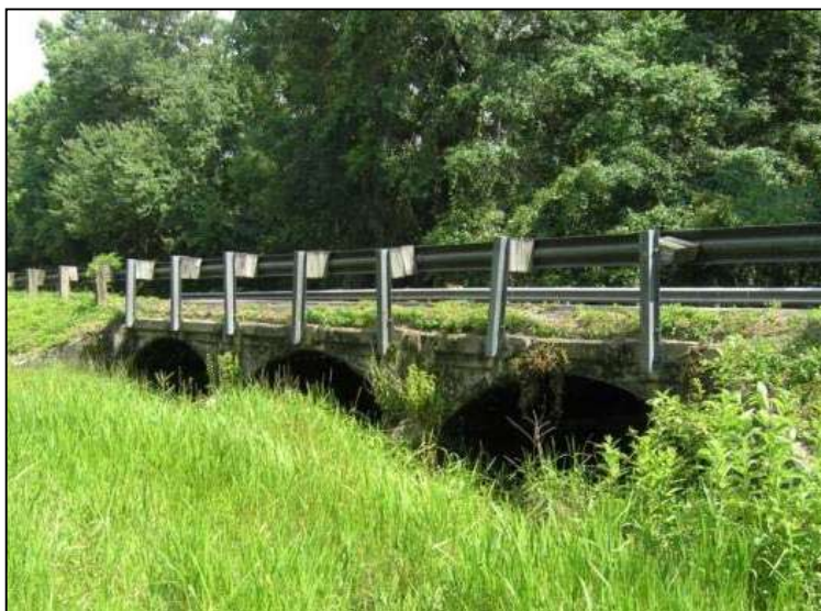
Photo 5-49. CR-18 over Gum Creek, Bradford County (No. 280037)
