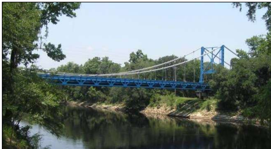
Photo 5-45. Hal Adams Bridge, Lafayette County (No. 330009)
