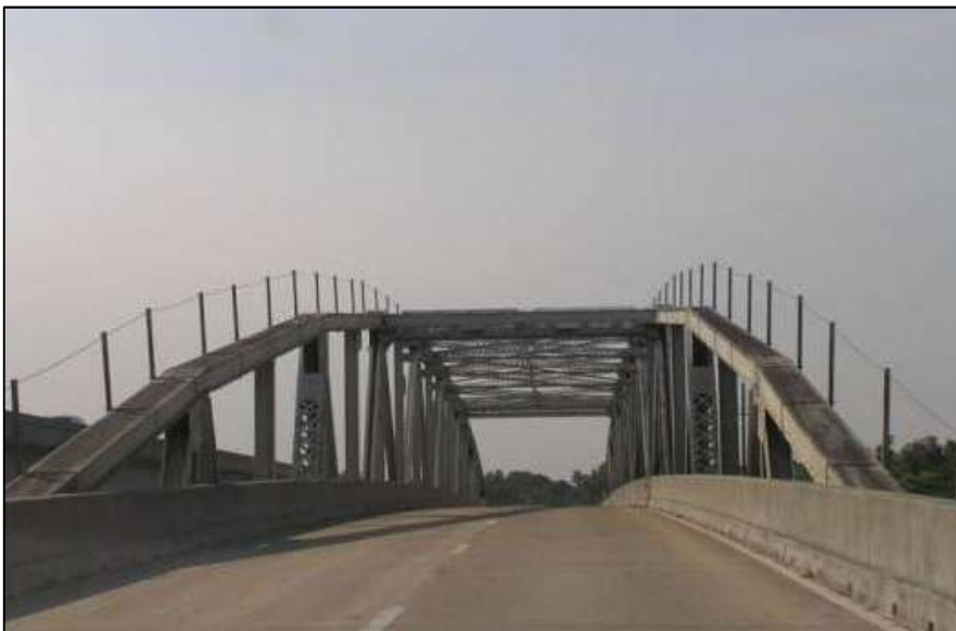
Photo 5-2. Blountstown Truss Bridge, Calhoun County (No. 470029)
