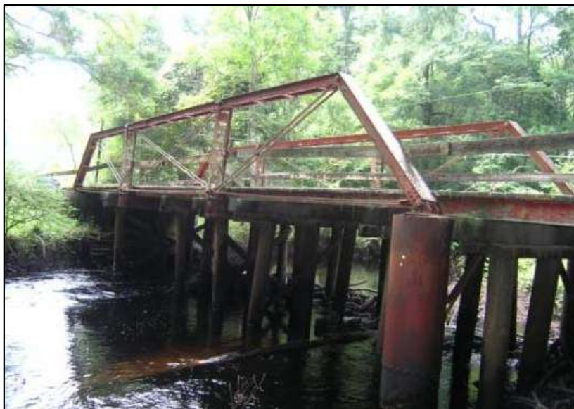
Photo 5-1. Steinhatchee Springs Bridge, Lafayette County (No. 334001)
