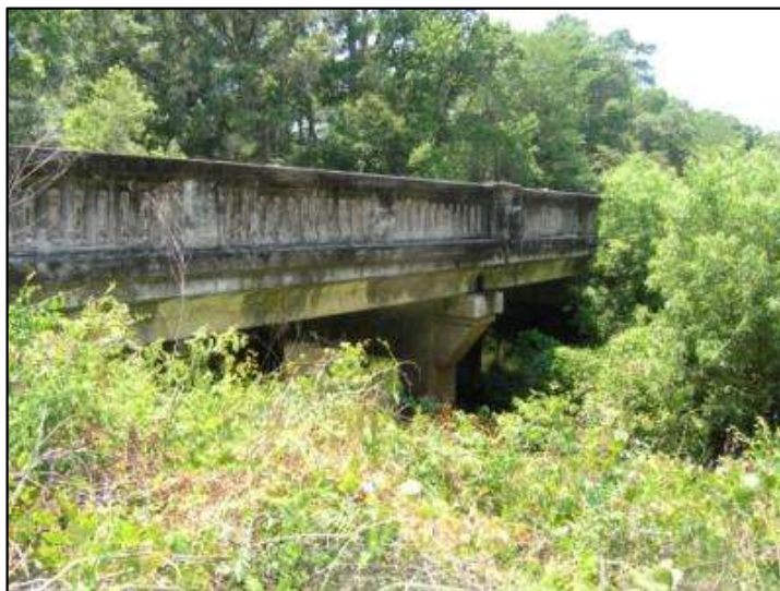
Photo 5-29. Ten Mile Creek Bridge, Levy County (No. 340045)
