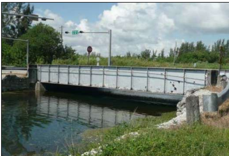
Photo 5-44. SW 117 th Avenue Bridge, Miami-Dade County (No. 874307)
