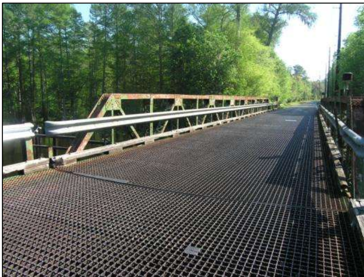
Photo 5-61. Sharpe's Ferry Swing Bridge, Marion County (No. 364110)
