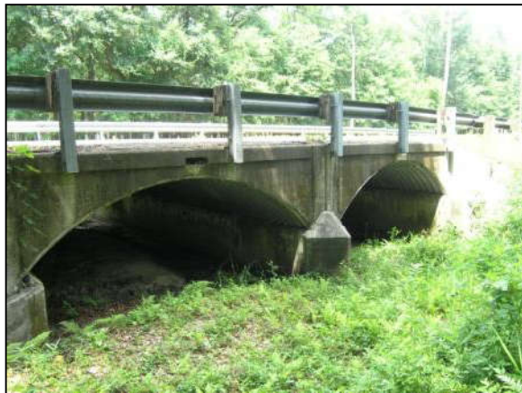
Photo 6-21. CR-18/Sampson River Branch Culvert, Bradford County (No. 280038)
