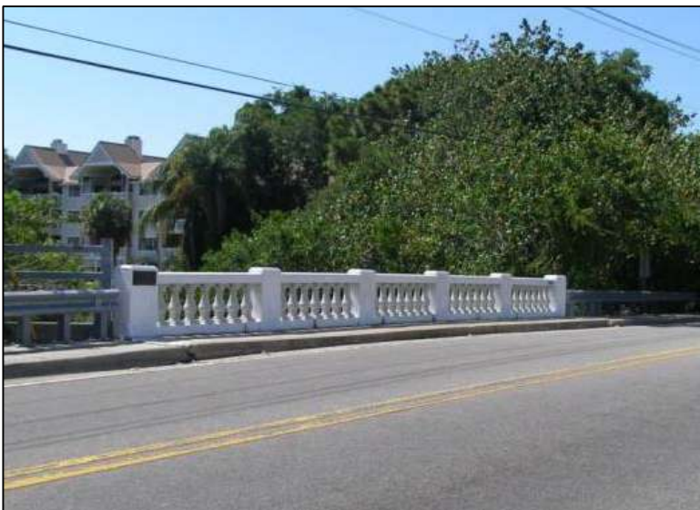
Photo 5-6. Osprey Avenue Bridge, Sarasota County (No. 175950)
