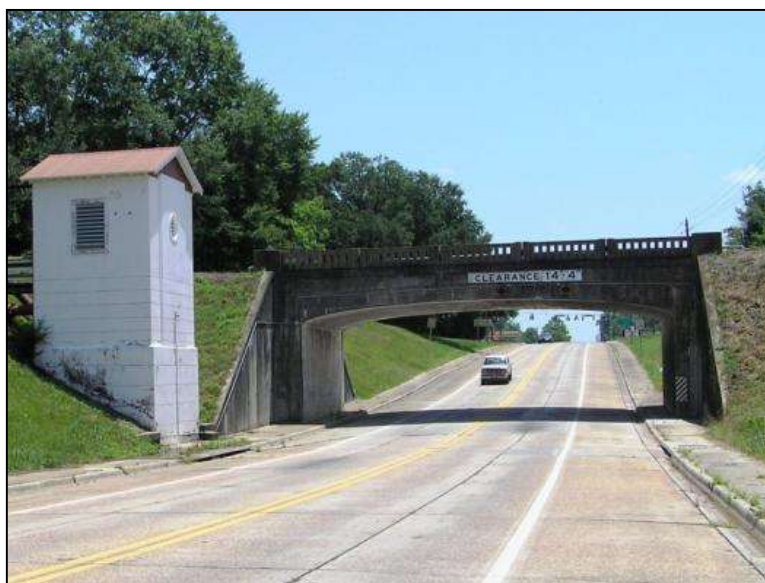
Photo 5-21. Atlanta and St. Andrews Bay Railway Frame Bridge, Jackson County (No. 530003)
