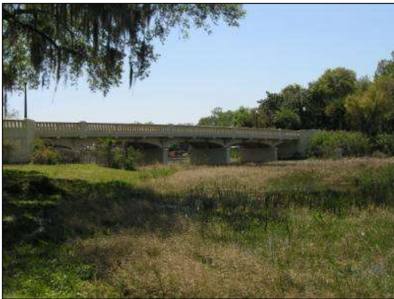
Photo 5-32. Lake Conway Bridge, Orange County (No. 755100)
