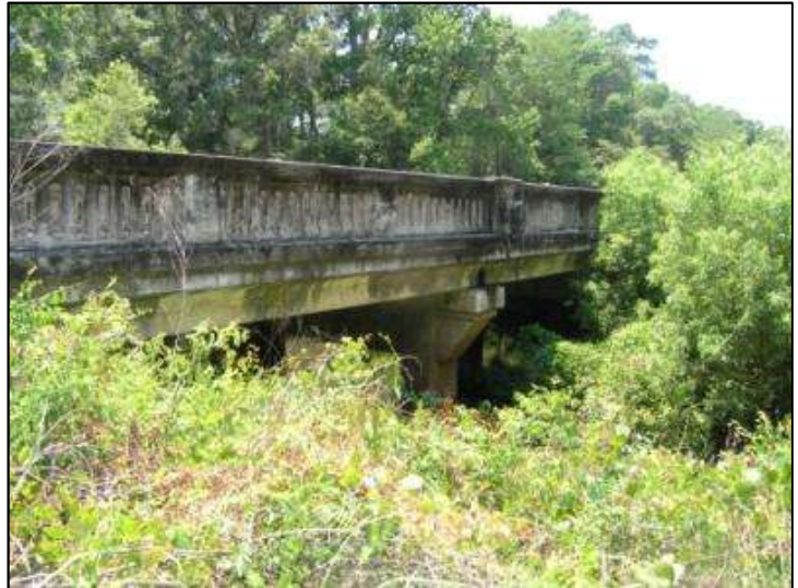
Photo 5-29. Ten Mile Creek Bridge, Levy County (No. 340045)
