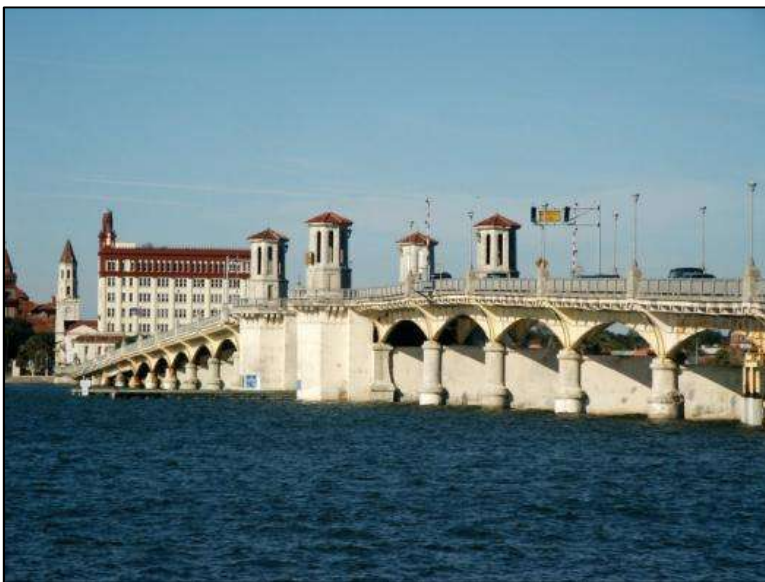
Photo 5-67. Bridge of Lions, St. Johns County (No. 780074)
