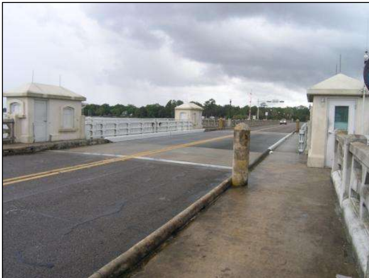
Photo 5-65. Ortega River Bridge, Duval County (No. 720005)
