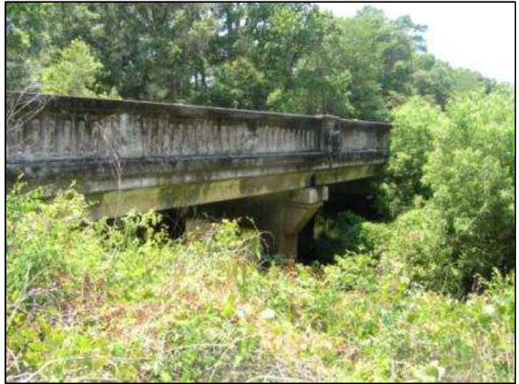
Photo 5-29. Ten Mile Creek Bridge, Levy County (No. 340045)
