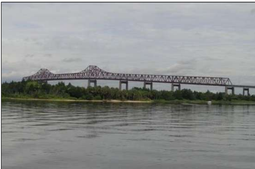
Photo 5-3. Mathews Bridge, Duval County (No. 720076)
