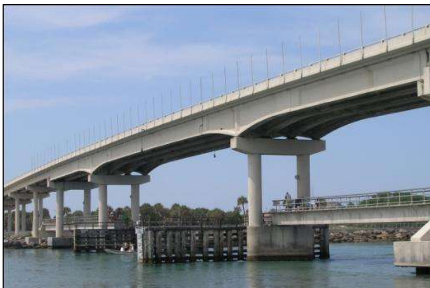
Photo 5-42. SR-A1A over Sebastian Inlet, Indian River County (No. 880005)
