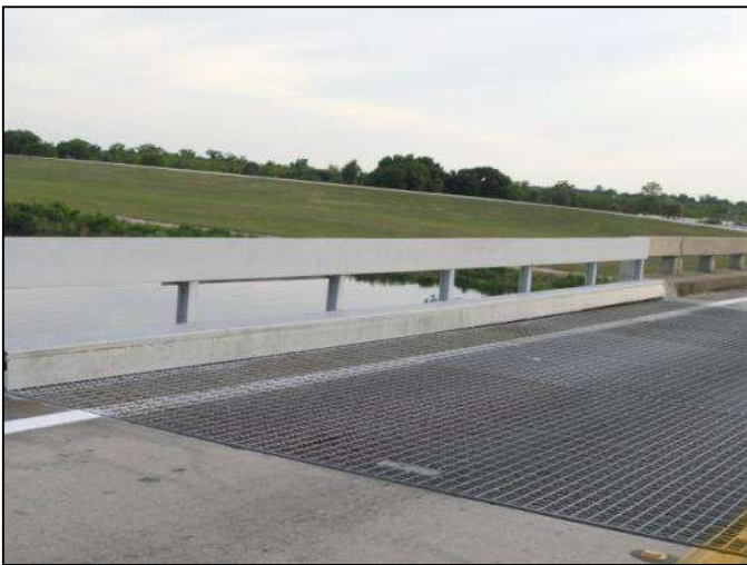
Photo 5-39. SR-78 Bridge (No. 910009) - Removable Span
