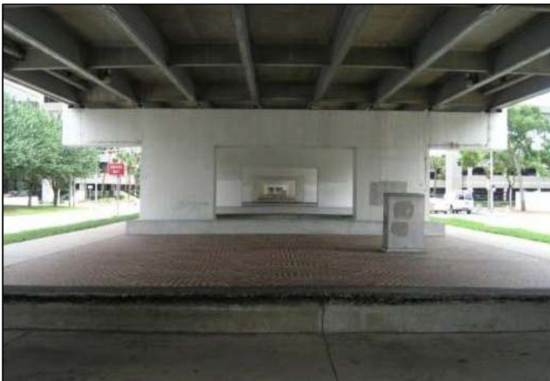
Photo 5-41. Plaza beneath Bridge No. 720087, Duval County
