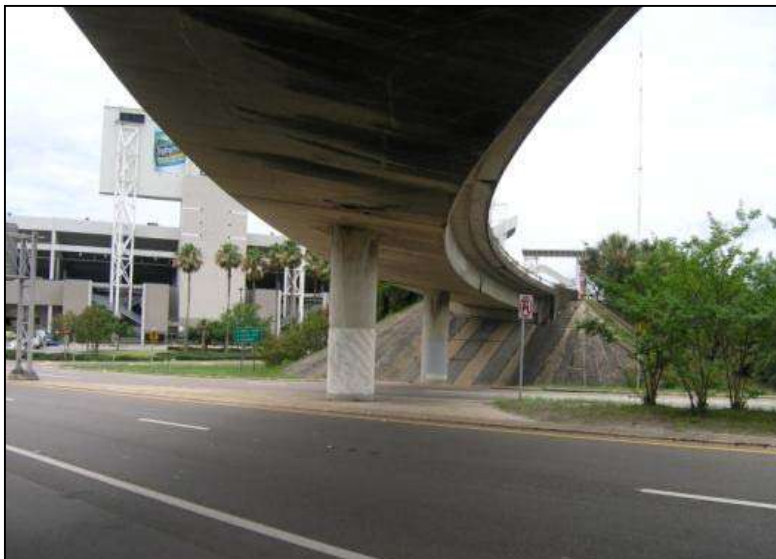
Photo 5-36. SR-115A Flyover to SR-10A, Duval County (No. 720100)
