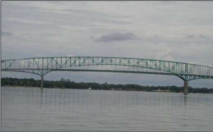
Photo 5-4. Hart Bridge, Duval County (No. 720107)
