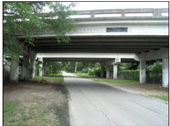
Photo 6-32. SR-228 at Ryar Road Prestressed Concrete Girder Bridge Pair (Nos. 720112/720283)
