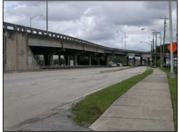
Photo 6-30. SR-228 at US-90 Steel Girder Bridge (No. 720113)
