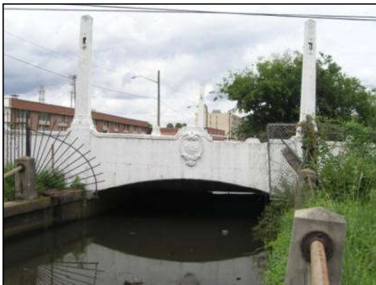
Photo 6-13. Market Street Bridge (No. 724172)
