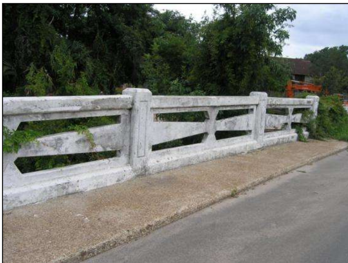
Photo 5-27. Myrtle Avenue Bridge, Duval County (No. 724258)
