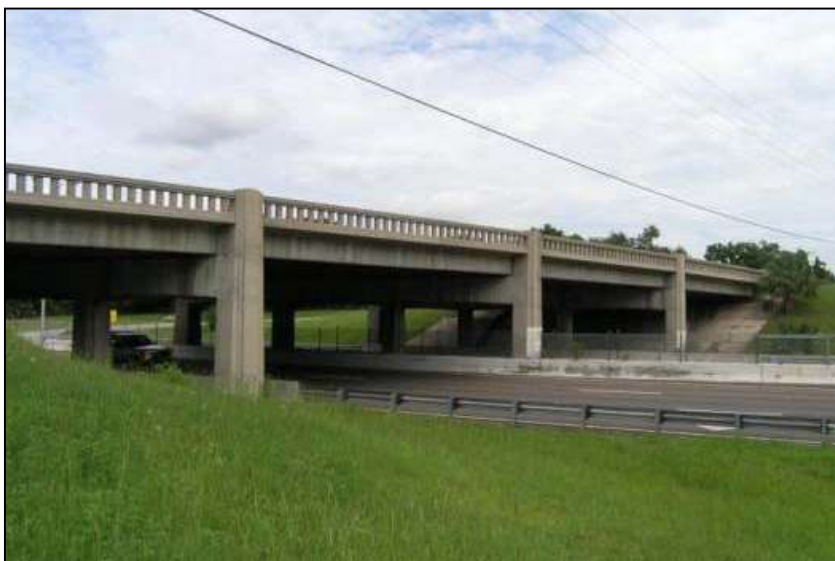
Photo 5-28. SR-109/University Avenue over SR-10A, Duval County (No. 720075)
