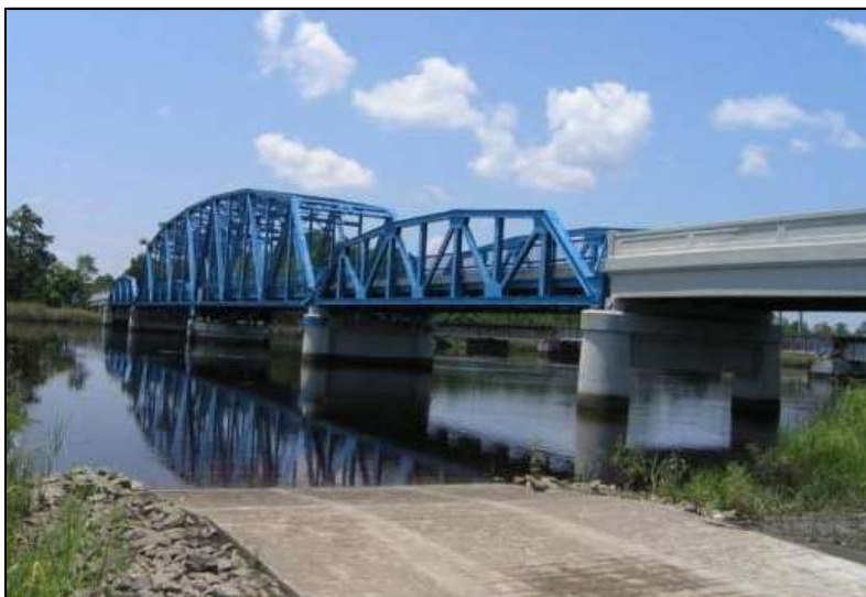
Photo 5-57. St. Mary's River Swing Bridge, Nassau County (No. 740008)
