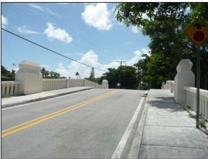
Photo 5-15. Seybold Canal Bridge, Miami-Dade County (No. 876500)
