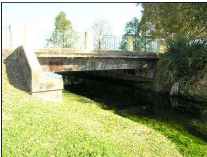
Photo 5-31. Poinsettia Avenue Bridge, Orange County (No. 755807)
