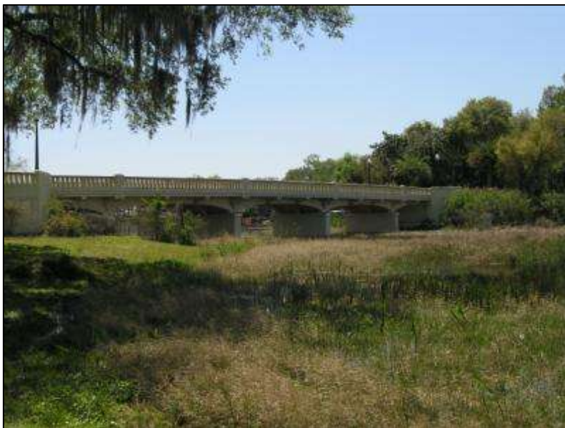
Photo 5-32. Lake Conway Bridge, Orange County (No. 755100)
