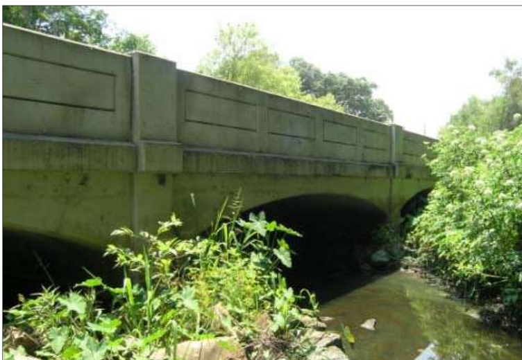
Photo 5-10. Old San Mateo Road Bridge, Putnam County (No. 764024)
