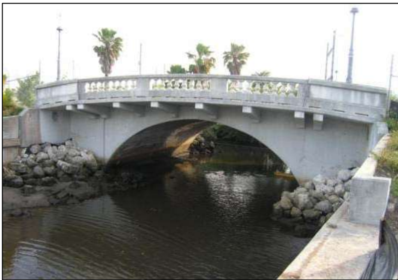
Photo 5-11. Moore's Creek Bridge, St. Lucie County (No. 945000)
