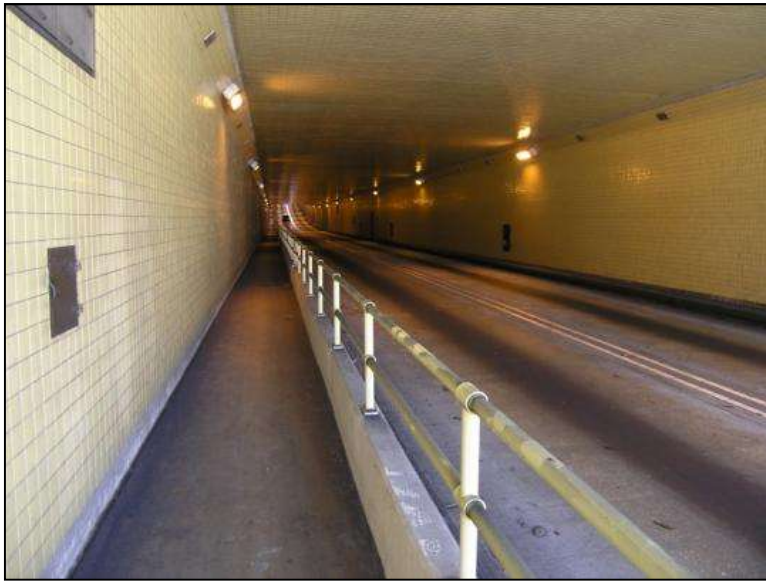
Photo 5-84. Henry Kinney Tunnel - Interior, Broward County (No. 764039)
