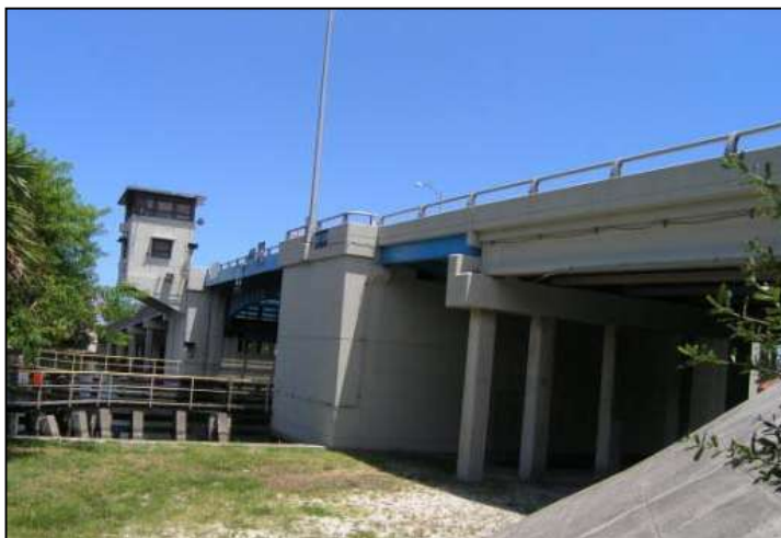
Photo 5-69. Davie Boulevard Bridge, Broward County (No. 860038)
