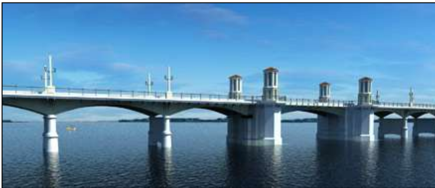
Photo 5-68. View of the Rehabilitated Bridge of Lions
