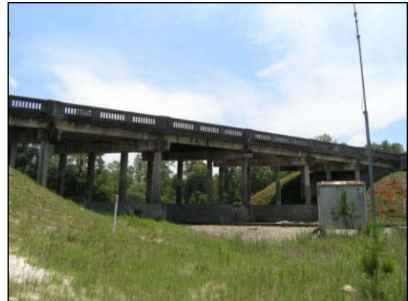
Photo 6-26. 1936 Sanderson Overpass, Baker County (No. 270001)
