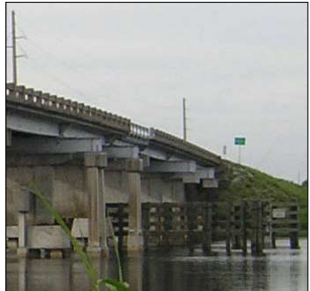
Photo 6-28. Bridge No. 090016 with Detail View of Removable Span.
