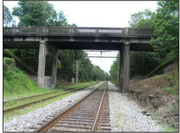
Photo 6-24. US-301/SR-200 over SCL RR, Nassau County (No. 740022)
