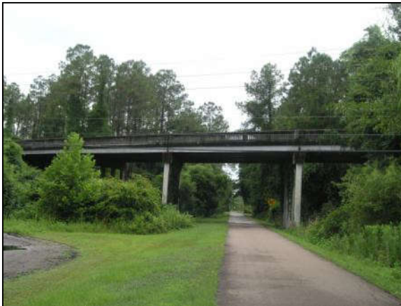
Photo 6-25. 1940 Baldwin Overpass, Duval County (No. 720026)
