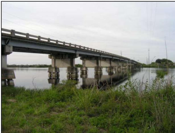
Photo 6-27. US-90 (SR-700) Bridge over the Kissimmee River, Highlands County (No. 090016)
