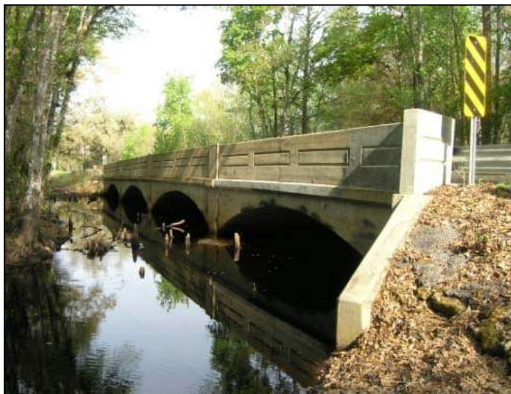
Photo 5-13. Deep Creek Arch Deck, Volusia County (No. 794081)
